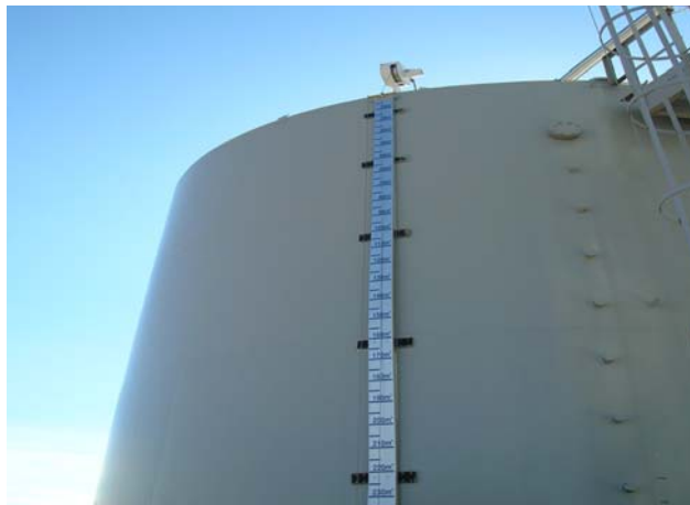
Redtail Hawk level gauge head with Goshawk transmitter
