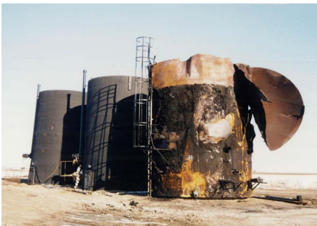
Tank that was over pressured due to inadequate vapor control.
