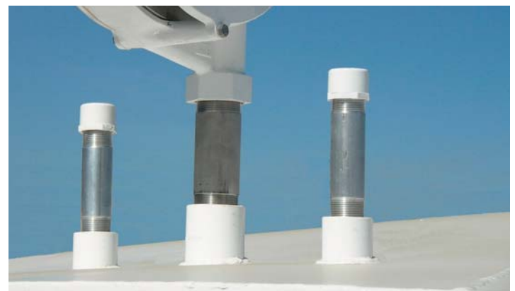
Above: Spring cable tensioners installed on a tank Below: Drop-in anchor plate.
